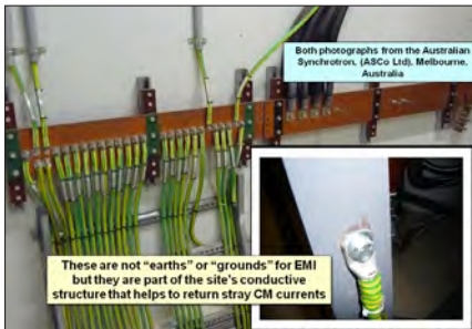
Figure 12. These are not “earths” or “grounds” for SI, PI or EMI either.
